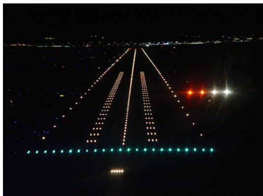
Obr. 17 – Precision Approach Path Indicator
