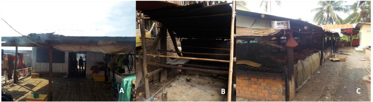
Figure 16 Three representatives of traditional smokehouse in Tonle Sap area, Cambodia, A – metal sheet smokehouse, B – wooden smokehouse, C – brick smokehouse with metal roof.
