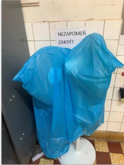
Figure 13: Unnecessary fans in winter
