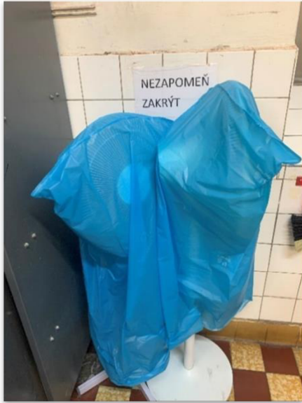
Figure 13: Unnecessary fans in winter
