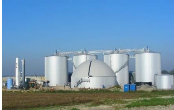
Fig 8. Example of industrial biogas plants in Netherlands (Krieg & Fisher-Ingenieure GmbH, 2011)
