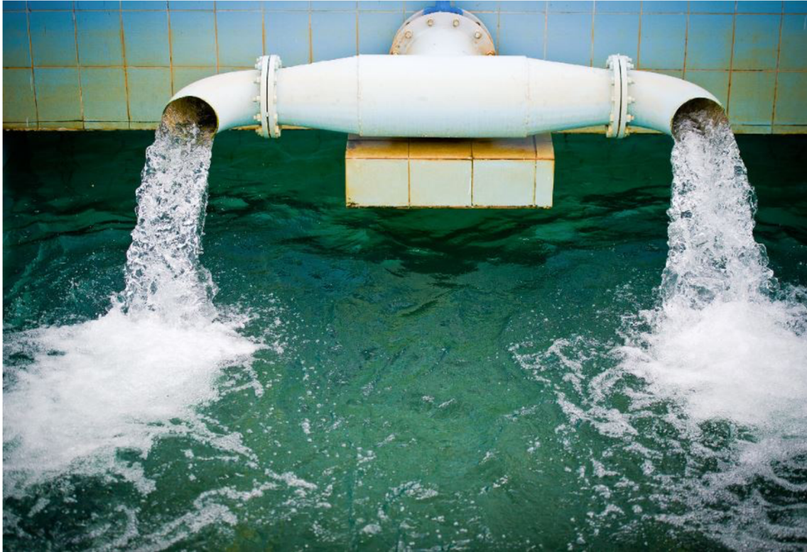
Figure 6 Sunyani water supply extension project in Ghana to commence
