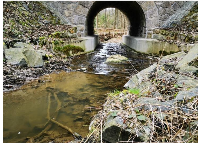
FIGURE 25: Existing location for the outlet hole, Photo taken by Author
