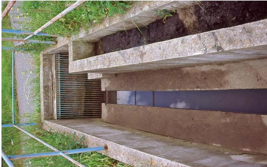
FIGURE 11: Screens and sand trap in Kámen u Havlíčkova Brodu. Photo credit: Jan Vymazal. Source: (Vymazal, 2004)
