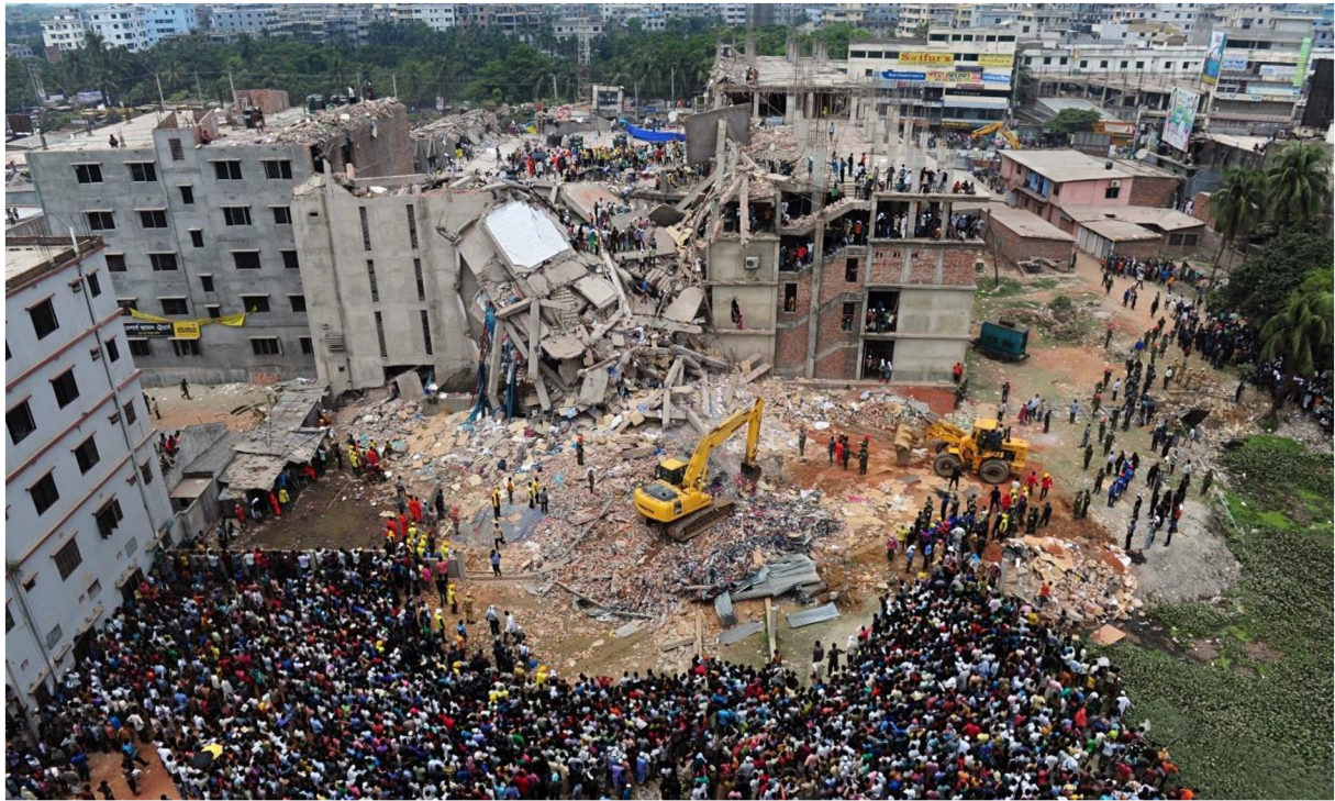
Figure 4: Aerial view of the Rana Plaza building site after it collapsed in April 2013
