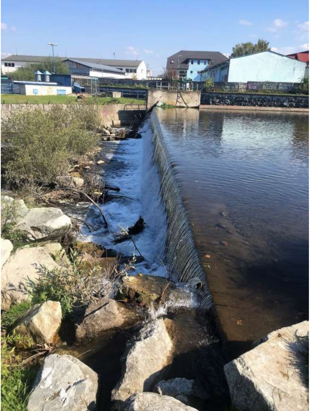
Picture 12. Two-meter high weir shortly after the beginning of RE07 section
