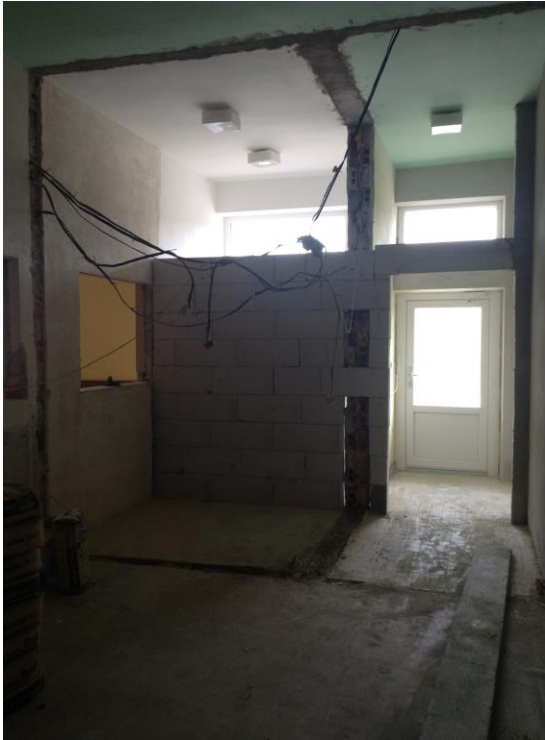
Fig. 54: The interior of changing room in construction 1
