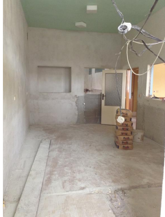
Fig. 55: The interior of changing room in construction 2
