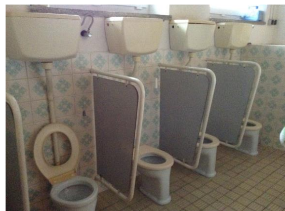
Fig. 32: An earlier condition 4
