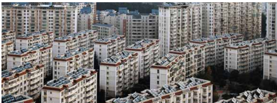
Obr. 404: Chenggong District, Kunming, Yunnan
