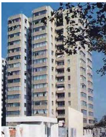
Obr. 294–295: Aijian Building, Šanghaj
