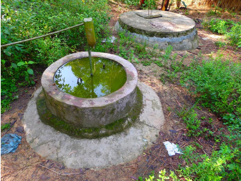
Figure 4 Small-scale biogas plant in Vietnam.
