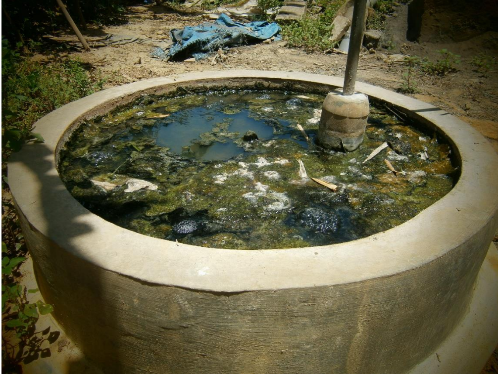
Figure 5 Small-scale biogas plant in Vietnam with leakages.
