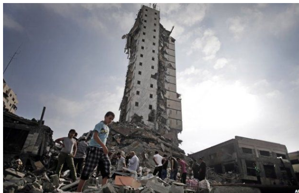
Example 6: The strike on the Italian Complex - which contained about 50 flats - caused one side of the tower to collapse
