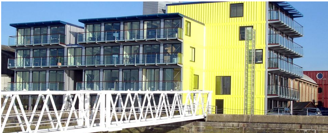
Obr. 3.9: The Riverside Building, Londýn, 2005 [32]
