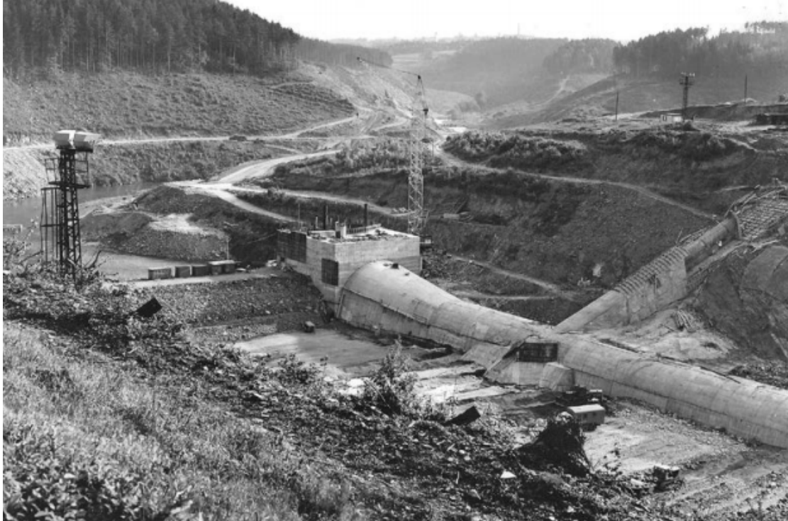
G. The Římov Reservoir – construction of the dam, 1974–1975. (Source: Znachor, P et al 2016).
