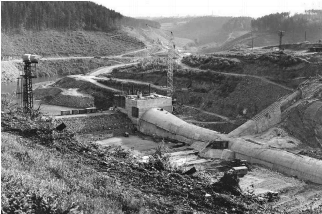
G. The Římov Reservoir – construction of the dam, 1974–1975. (Source: Znachor, P et al 2016).
