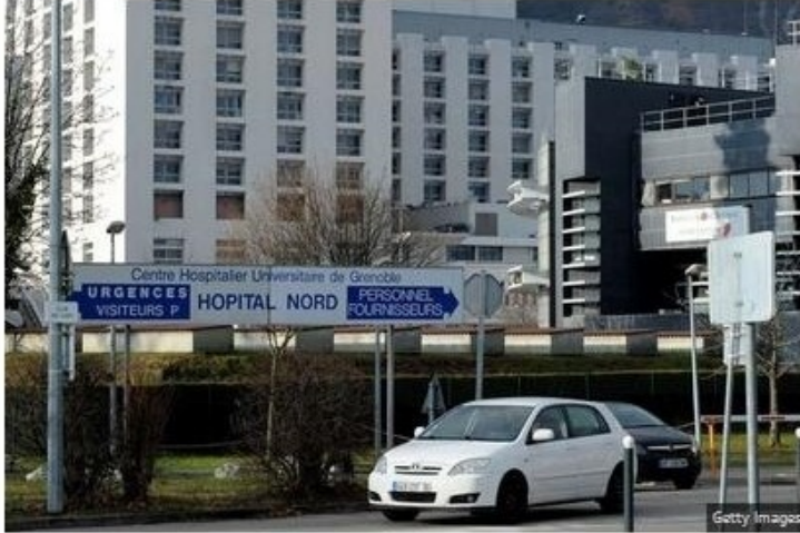
Hospital: Centre Hospitalier Universitaire In Grenoble
