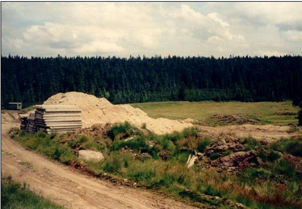
Figure 27: Pile of sand and concrete panels at former Roklan reservoir. 1991 ©Zdeněk Uher.
