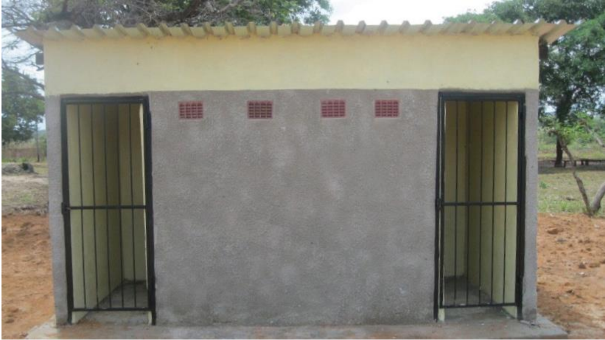
Image 2. ZWASH project constructed VIP Latrine 65
