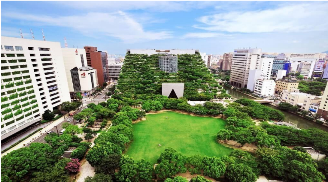
Figure 7 ACROS Fukuoka Prefectural International Hall (source: greenroofs.com, 2017)
