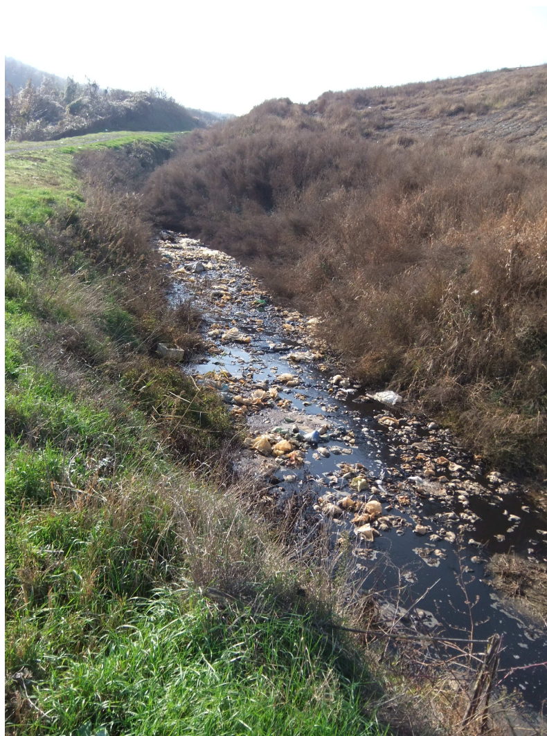
Photo 12. – Wastewater with no treatment at Vinca Landfill
