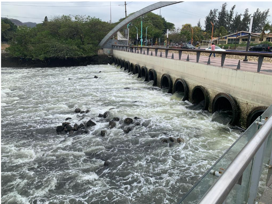
Figure 2.2: Photograph of the downstream side of Urdesa bridge and its flood control valves. Photo taken by Luis Dominguez.
