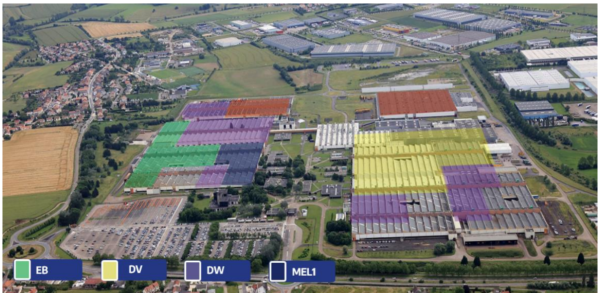
Figure 2.2.2 the Trémery plant with the breakdown by sector of activity[27].
