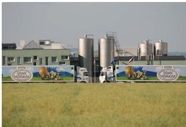
Figure 5.1 Facility of Company Orrero a.s, Tři Dvory 98, source Orrero
