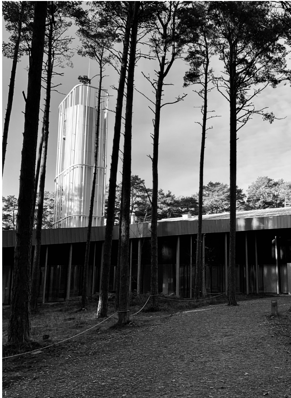
1. Estonia, Arvo Part Centre. Photo by: Nikita Akindinov. Oct 2020 2. Estonia, Arvo Part Centre. Aerial view. Image by: Roland Halbe. Source: https://www.designcurial.com/news/part-of-the-landscape-arvo-part-centre-by-nieto-sobejano-6909529/ , [ accessed 09.04.2023 ]
