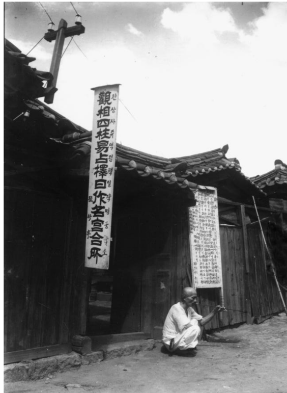
Figure 3 House of a fortune teller from colonial era. Source: National Museum of Korea.
