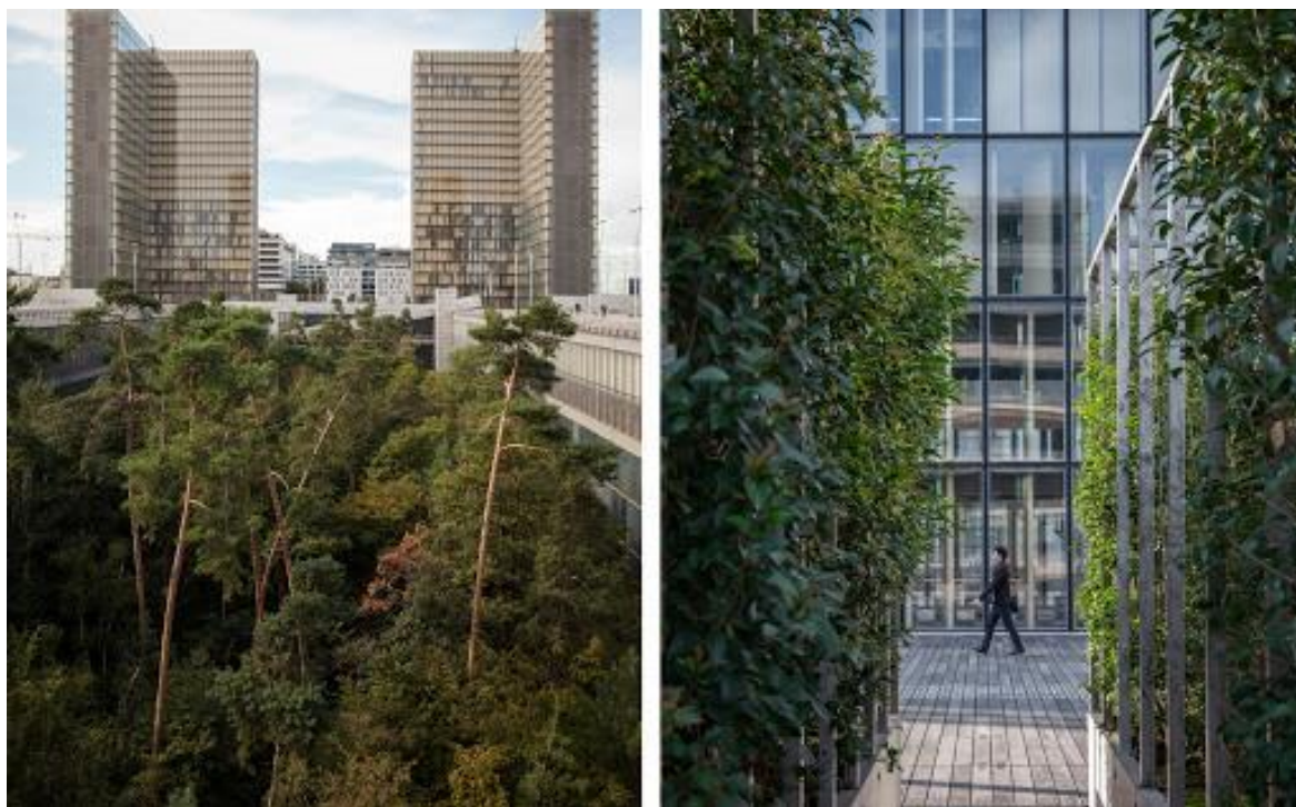
Obr. 11: Bibliothèque nationale de France (zdroj: http://architectuul.com/architecture/french-national-library )
