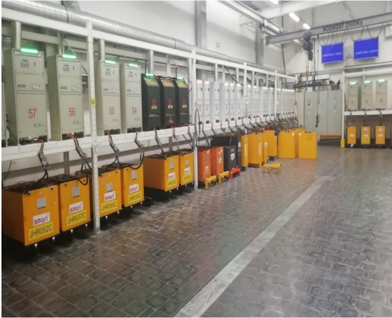
Figure 15: Charging station in Hall M2
