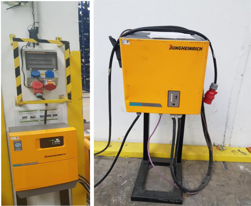
Figure 24: Chargers for Li-ion batteries (left – charger installed on the pillar, right – charger stand)
