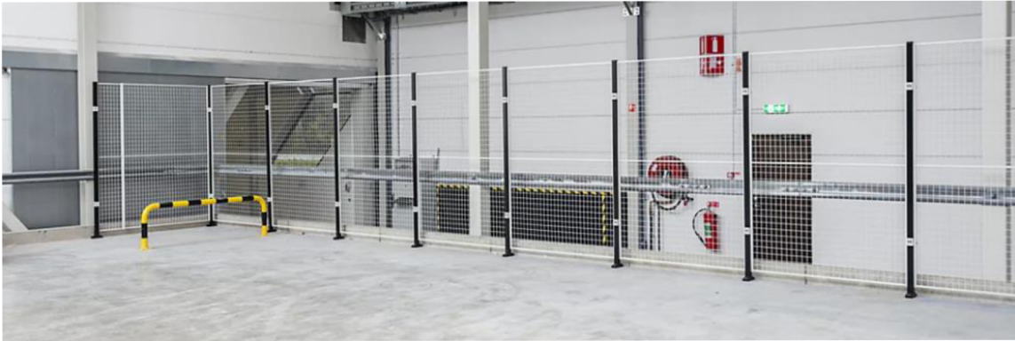
Figure 23: Proposed parking lot for handling equipment with Li-ion battery between pillars
