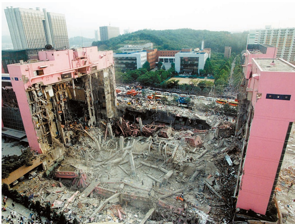
Obr. 2.7 Havárie budovy Sampoong Department Store, Soul, Jižní Korea [6]
