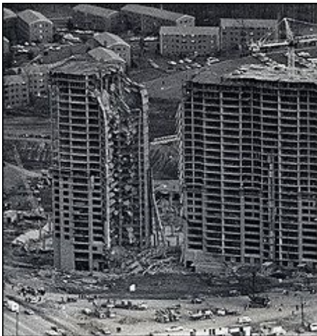
Obr. 2.5 Havárie budovy Skyline Plaza, Virginia, USA, 1973 [4]
