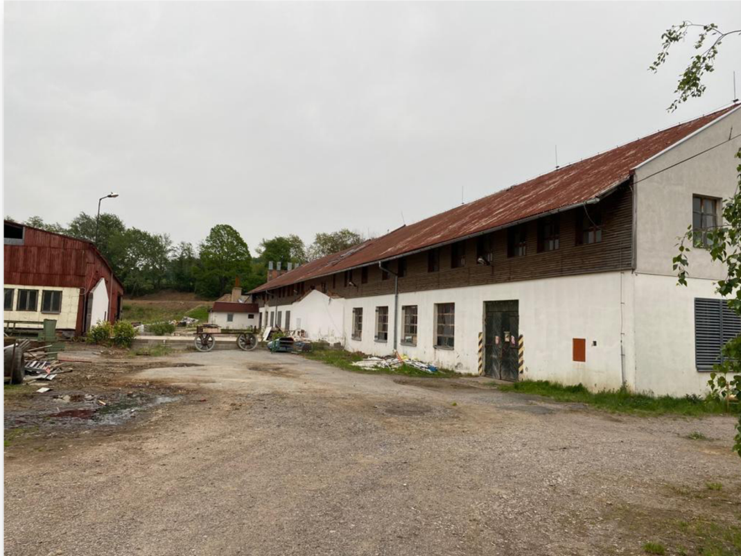
Figure 7, area for the warehouse prior to the construction
