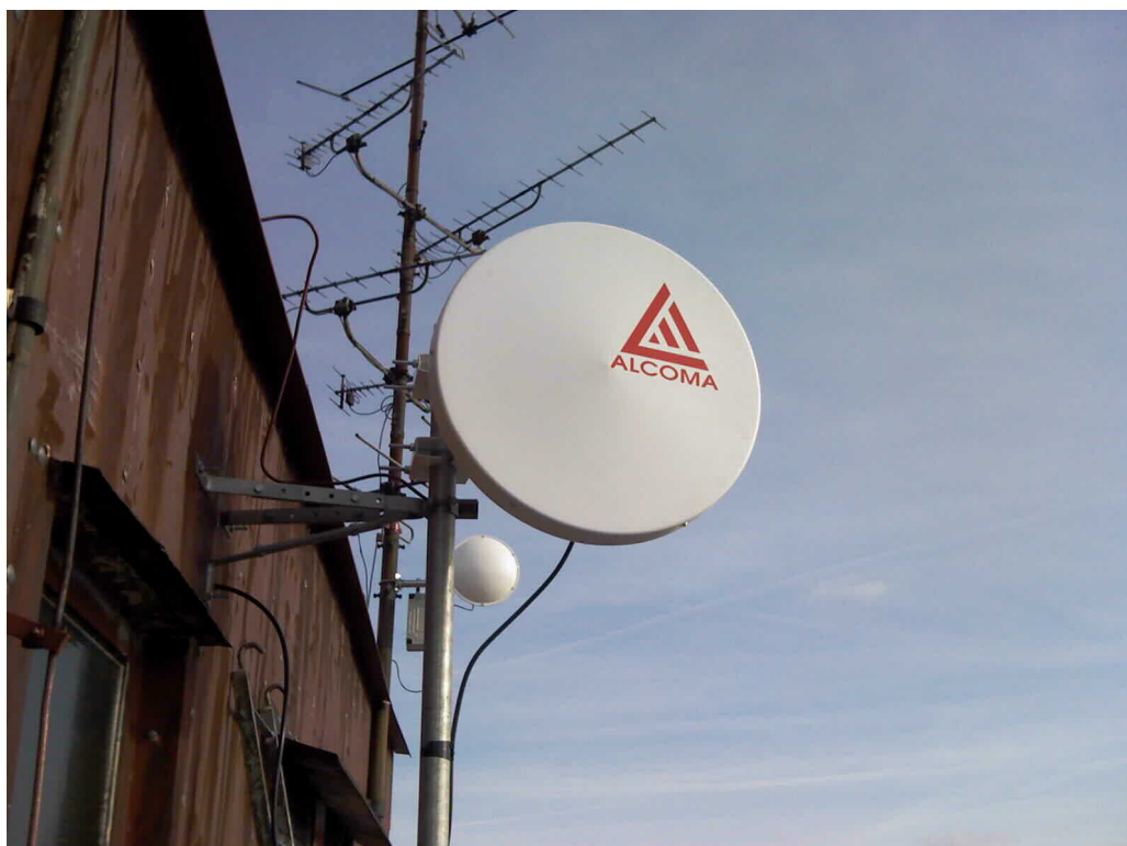
Obr. 17: Parabola 34 dB ALCOMA AL10F
