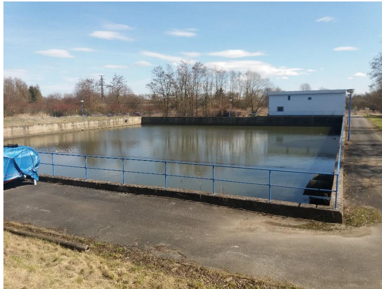
Fig. 19: Concrete retention tank – The retention tank collects water without providing any infiltration. The main intention was to reduce the stormwater runoff and regulate the outflow. (Photo by Author)
