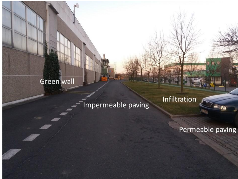
Fig. 15: The side view on the Standard site – The photo shows portion of impermeable surfaces and vegetation. (Photo by Author)
