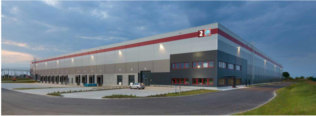
Fig. 2 – Archetypal view of large warehouse building with truck gates (docks) in left half of the building and manipulative impermeable area in front of them. Additionally, there is also a small parking lot in front of the office zone located in the right front corner of the building. (Photo and Copyright © 2018 Filson)
