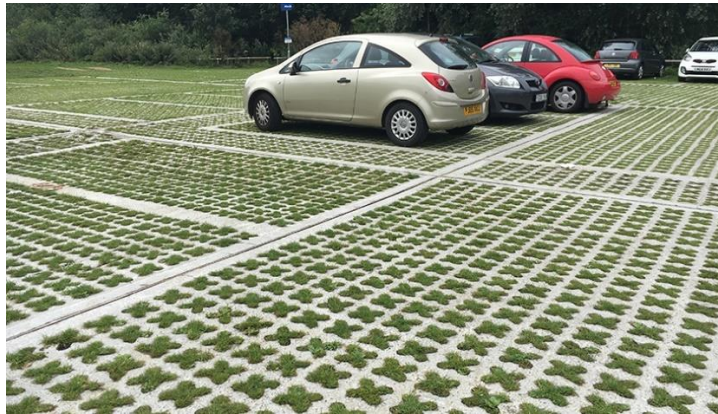
Fig. 28: Usage of grass concrete paving system - This photo demonstrates a usage of grass concrete paving system for parking lot (Photo by Grass Concrete Ltd.)
