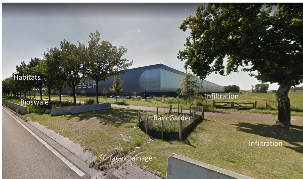
Fig. 24: Surroundings of the warehouse – Photo shows many opportunities for infiltrating the stormwater by green areas, enhanced by bioswale, rain garden or meadow in the background. (original picture from Google Maps)
