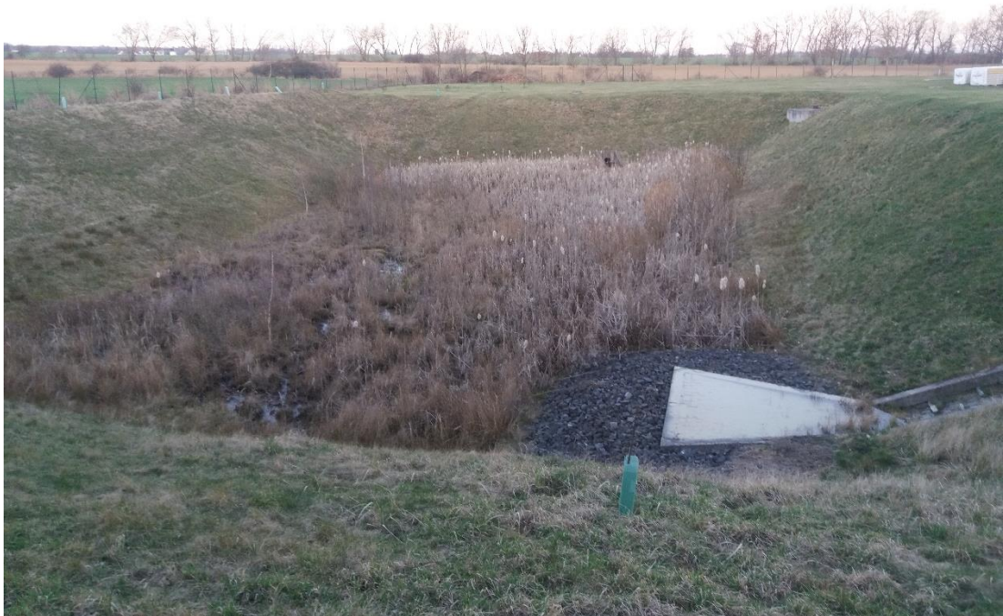
Fig. 15: Large infiltration basin – The photo present large infiltration basin that provides beside infiltration also habitats for local habitat, however only for small species due to fence around the site. (Photo by Author)
