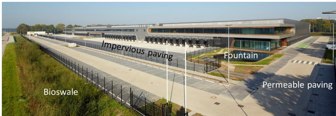
Fig. 22: Photo of the finished construction 09/2014 - Photo was taken, when the construction was finished (09/2014). You can see the front façade with main entrance, where you can see the infiltration basin with fountain in front of office part and the bioswale out of the fenced area in left part of the photo. (Photo by Dokvast; References – http://newlogicii.com/newlogic.php )
