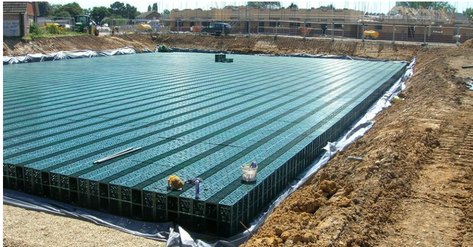
Fig. 37: Photo of stormwater infiltration blocks near South Coast of England - Individual blocks were put together, insulated with permeable textile and covered back with soil (Photo by Cole Easdon)
