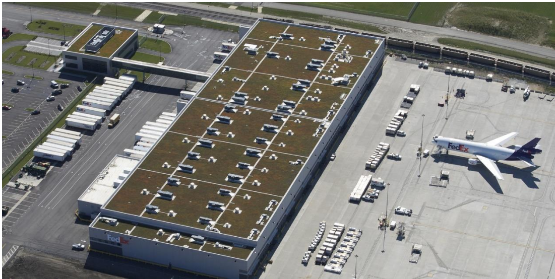
Fig. 30: O'Hare International Airport in Chicago - The FedEx has integrated green roof system on one of their facility at O'Hare International Airport in Chicago (Authors: Green Roof Solutions, Inc.; reference - http://www.greenroofsolutions.com/ )
