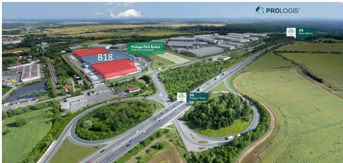
Fig. 17: Location plan of Prologis Park-Rudná next to the D5 highway with lighted Building 18 - middle blue as an original part and lateral red as an expansion part assessed as "Outstanding" with a final score 88,1% base on BREEAM accreditation (reference – Prologis Website)
