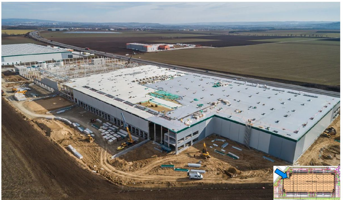
B.2/ PICTURE NO. 2 – STEEL CONSTRUCTION, FACADE, ROOF INSULATION
