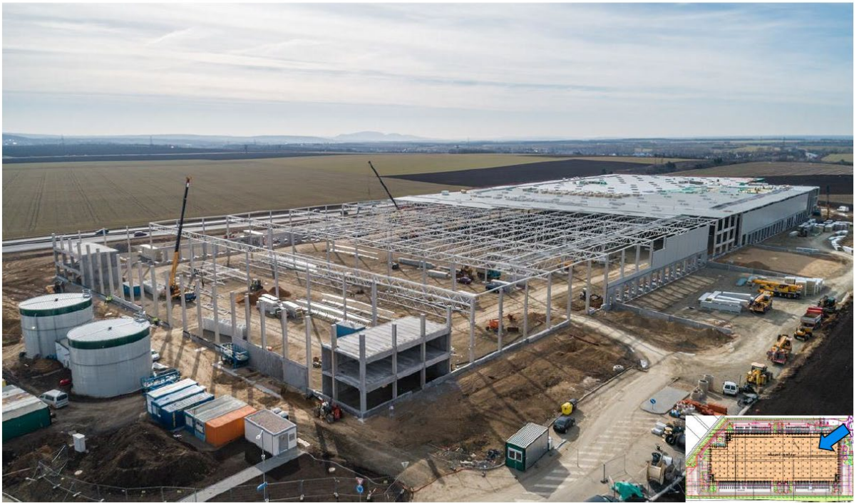
B.2/ PICTURE NO. 1 – STEEL CONSTRUCTION
