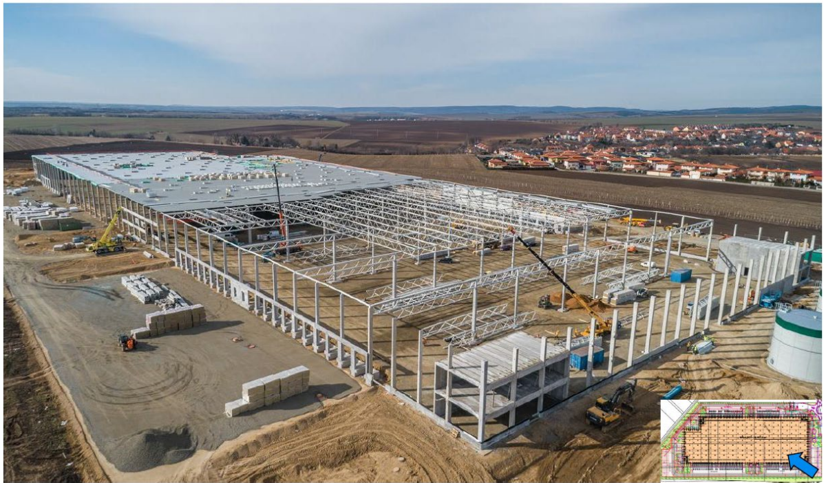
B.2/ PICTURE NO. 3 – STABILIZATION, STEEL CONSTRUCTION
