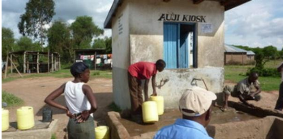
Figure 7 : Water kiosks in Kisumu slums
