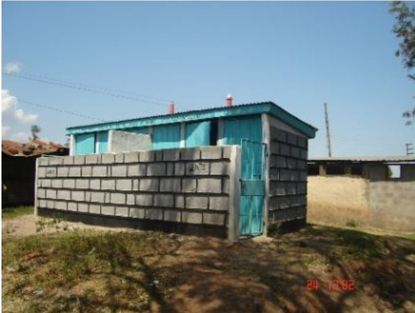
Figure 6 : Public toilets Otonglo Market Central Kisumu
