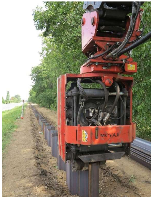
Figure 4.5 Steel Sheet pile wall construction (24)
