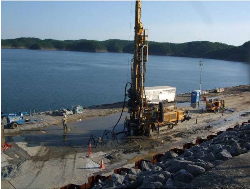
Figure 4.24 Application of cement grouting (29)
