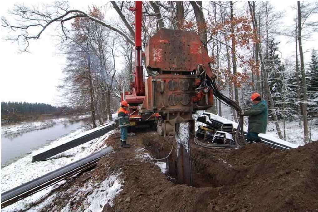
Figure 5.2 Construction of steel sheet pile wall (10)
