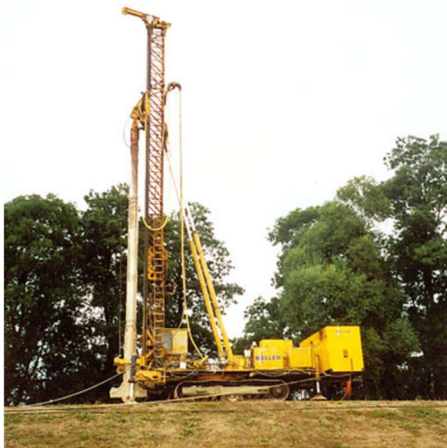
Figure 5.1 Work on cut-off wall (9)
