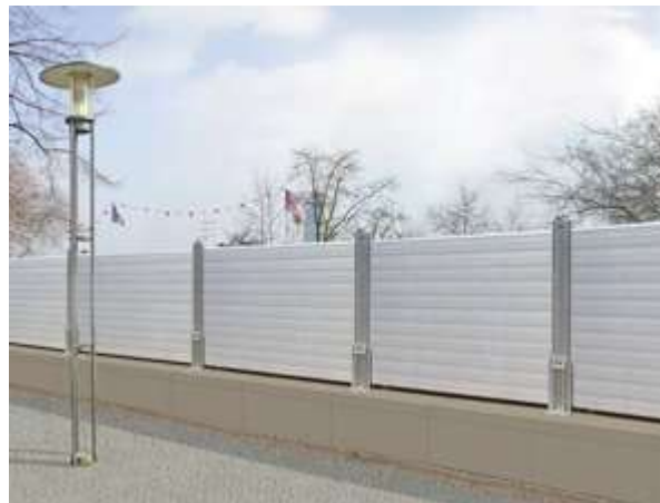
Figure 4.31 Raised Flood Wall (34)
