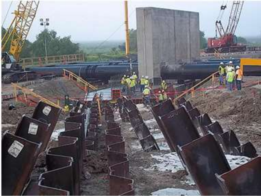
Figure 4.28 Driven piles prepared for T-wall (33)
