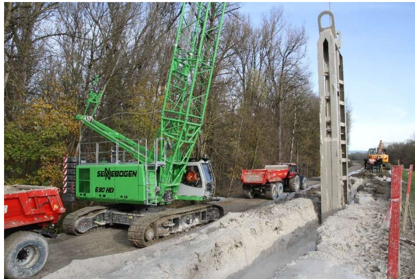
Figure 4.1 Work on diaphragm wall used for levee improvement (21)
