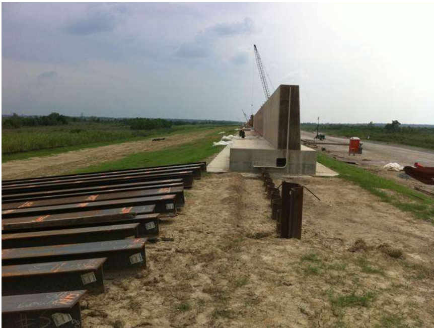
Figure 4.29 T-floodwall installation (35)
