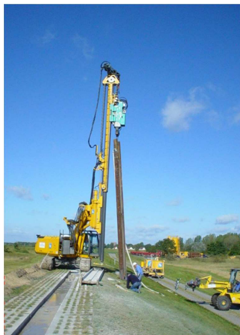
Figure 4.10 Construction of thin slurry wall (5)
