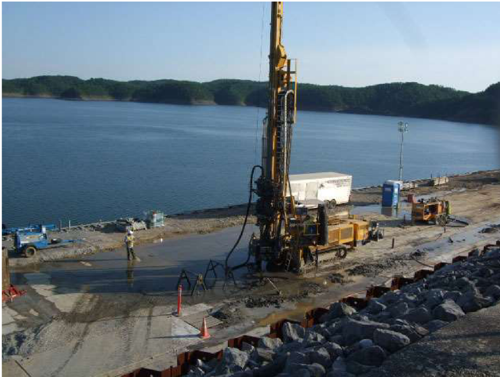
Figure 4.24 Application of cement grouting (29)
