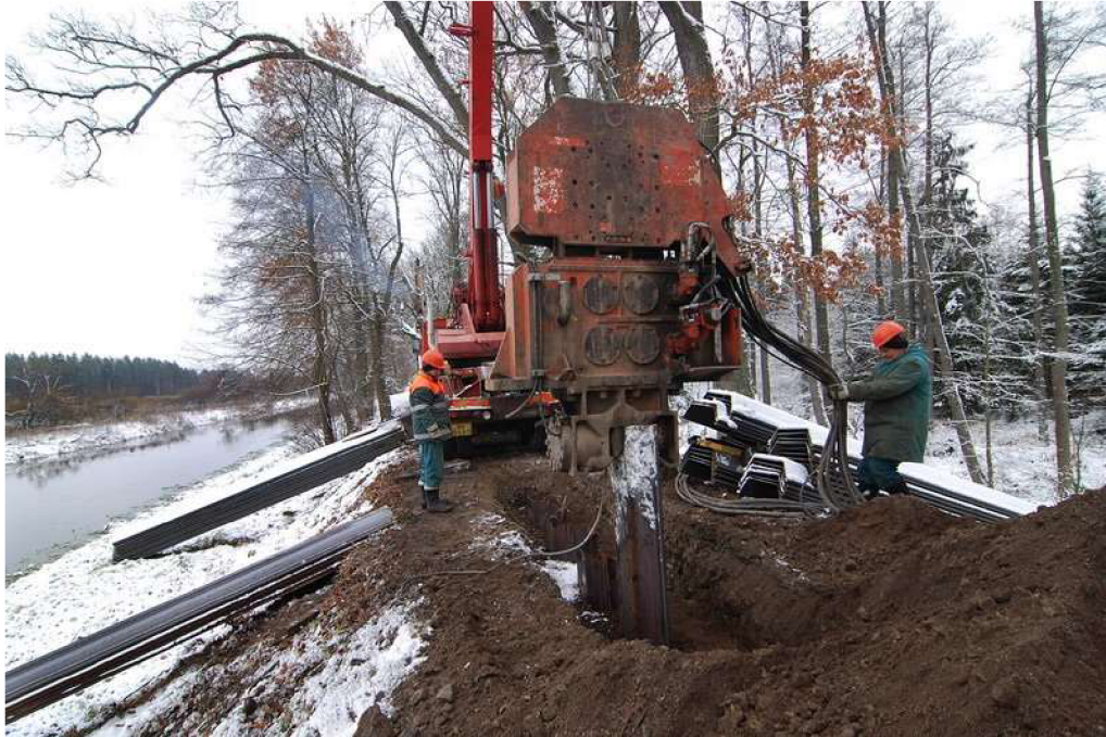
Figure 5.2 Construction of steel sheet pile wall (10)
