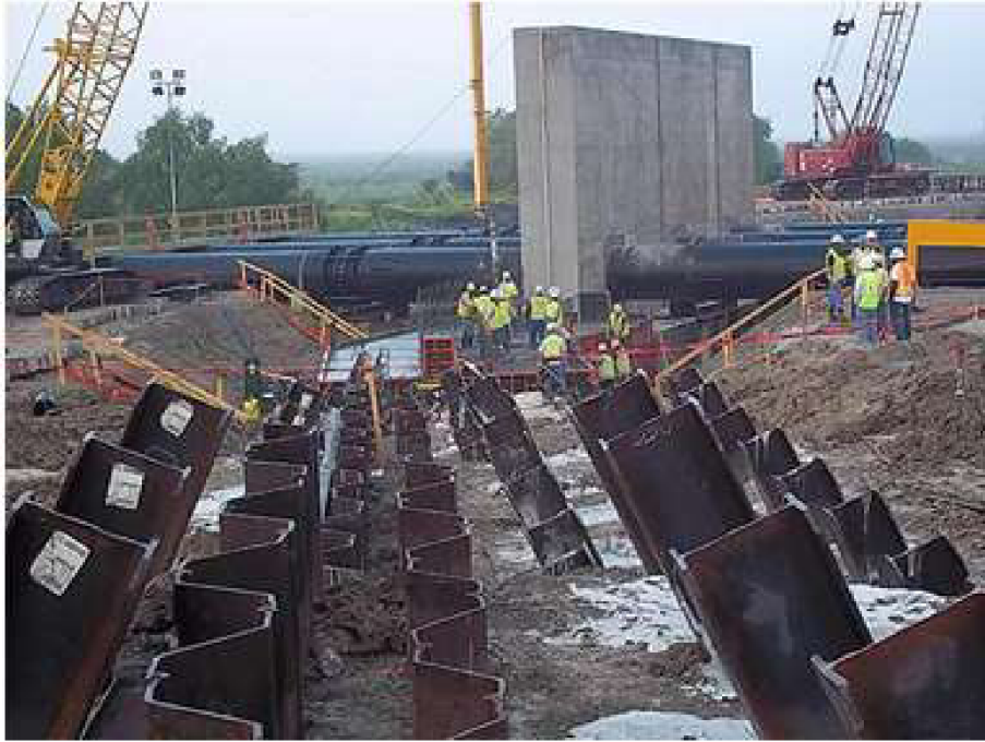
Figure 4.28 Driven piles prepared for T-wall (33)
