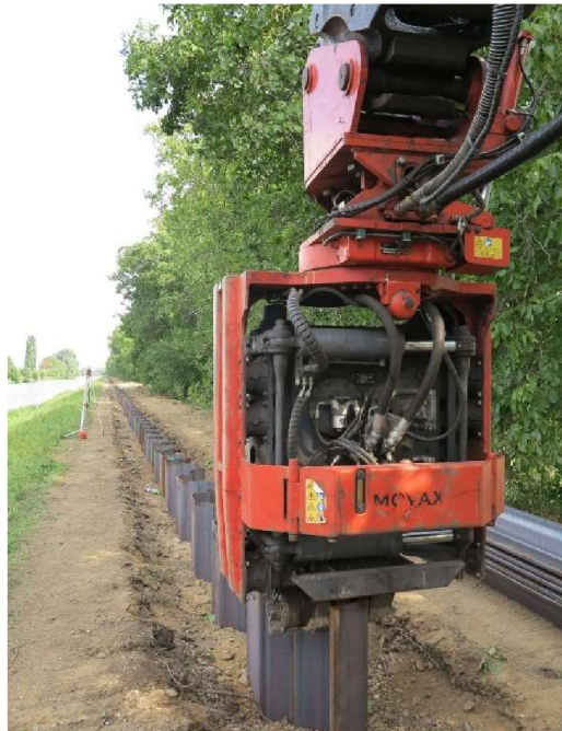
Figure 4.5 Steel Sheet pile wall construction (24)
