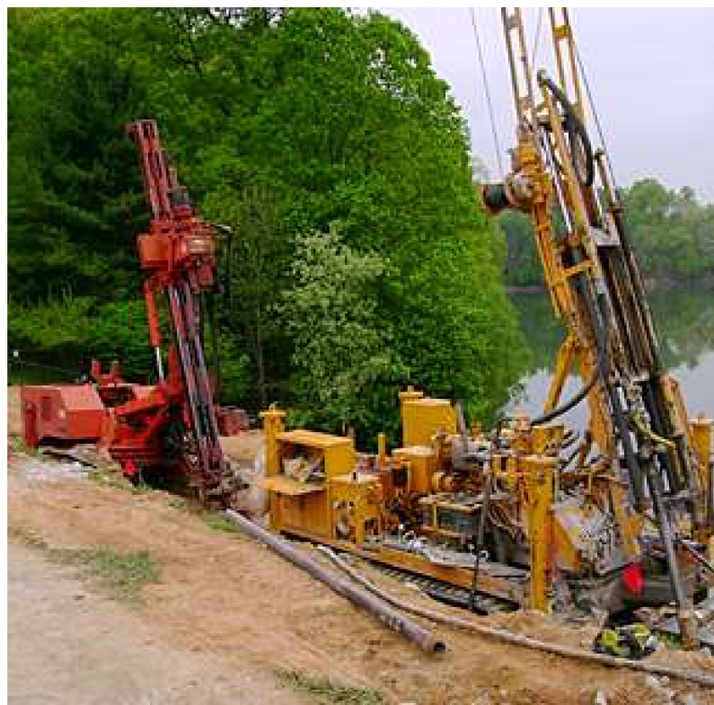
Figure 4.22 Jet Grouting (31)
