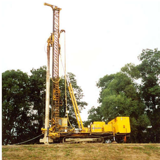
Figure 5.1 Work on cut-off wall (9)
