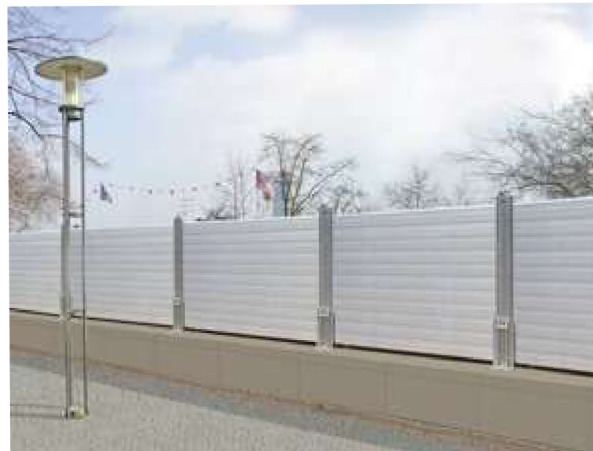
Figure 4.31 Raised Flood Wall (34)
