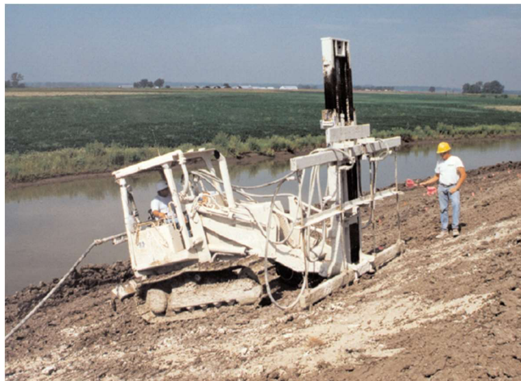
Figure 4.25 Injection stabilization (32)
