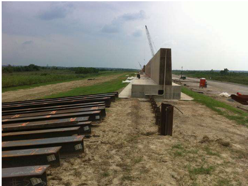
Figure 4.29 T-floodwall installation (35)
