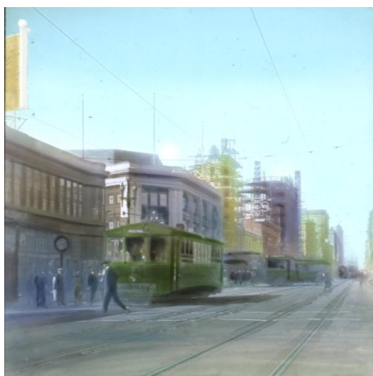
Market Street, San Francisco, USA, 1920-21.
