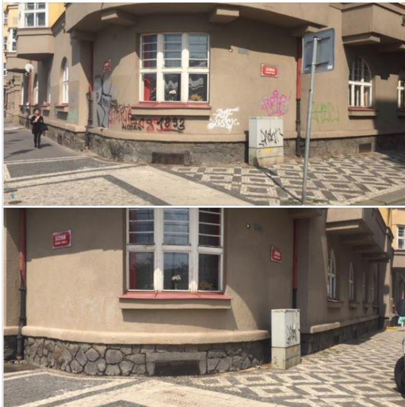
Figure 4.19: Showing a building restored from graffiti Source: (Antigraffiti program Prahy 3, 2018)
