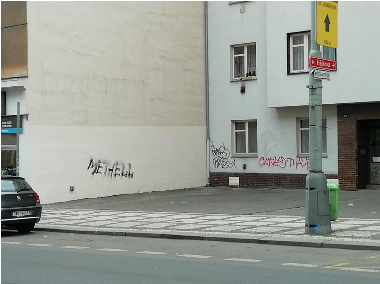
Figure 4.22: Showing a building cleaned with graffiti back on it
