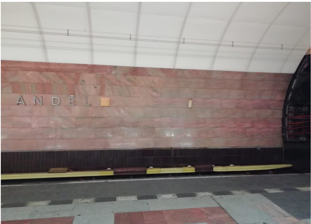
Figure 4.14: Showing the Andel metro station platform after clean up
