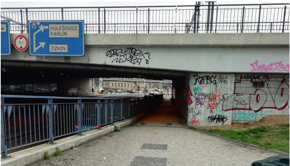
Figure 4.7: Showing graffiti under a bridge at Seifertova street, Prague 3
