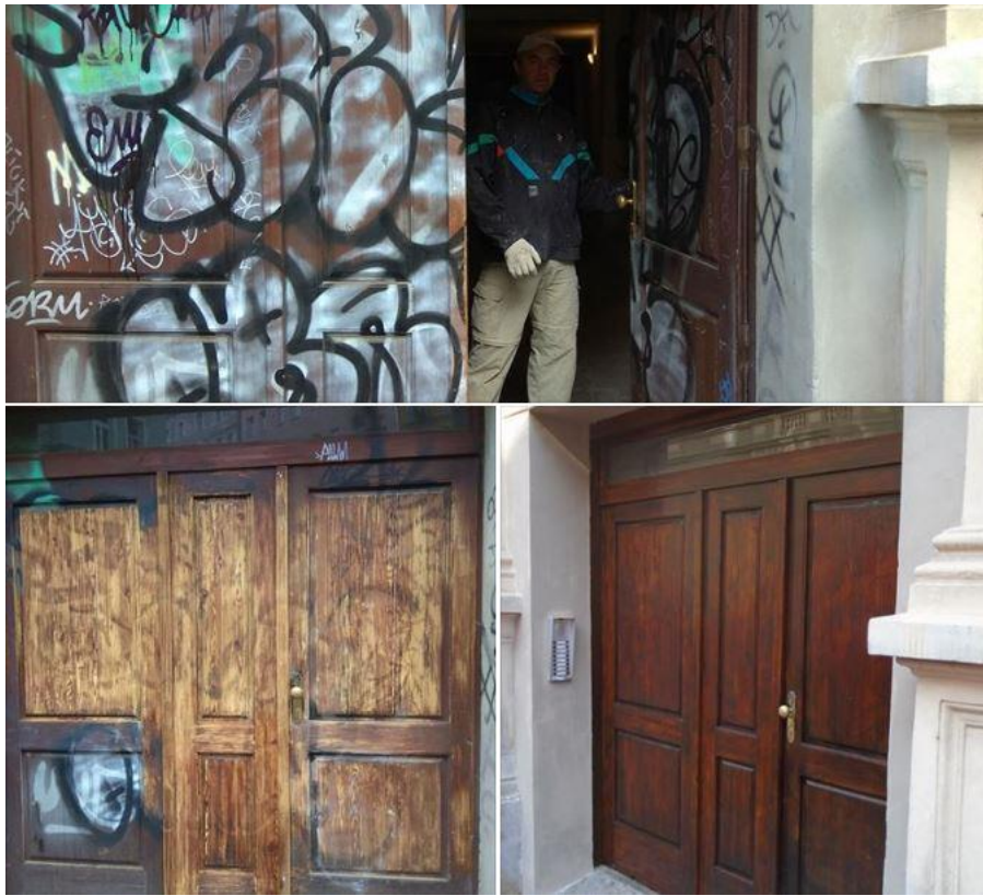
Figure 4.17: Showing a building restored from graffiti Source: (Antigrffiti program Prahy 3, 2018)
