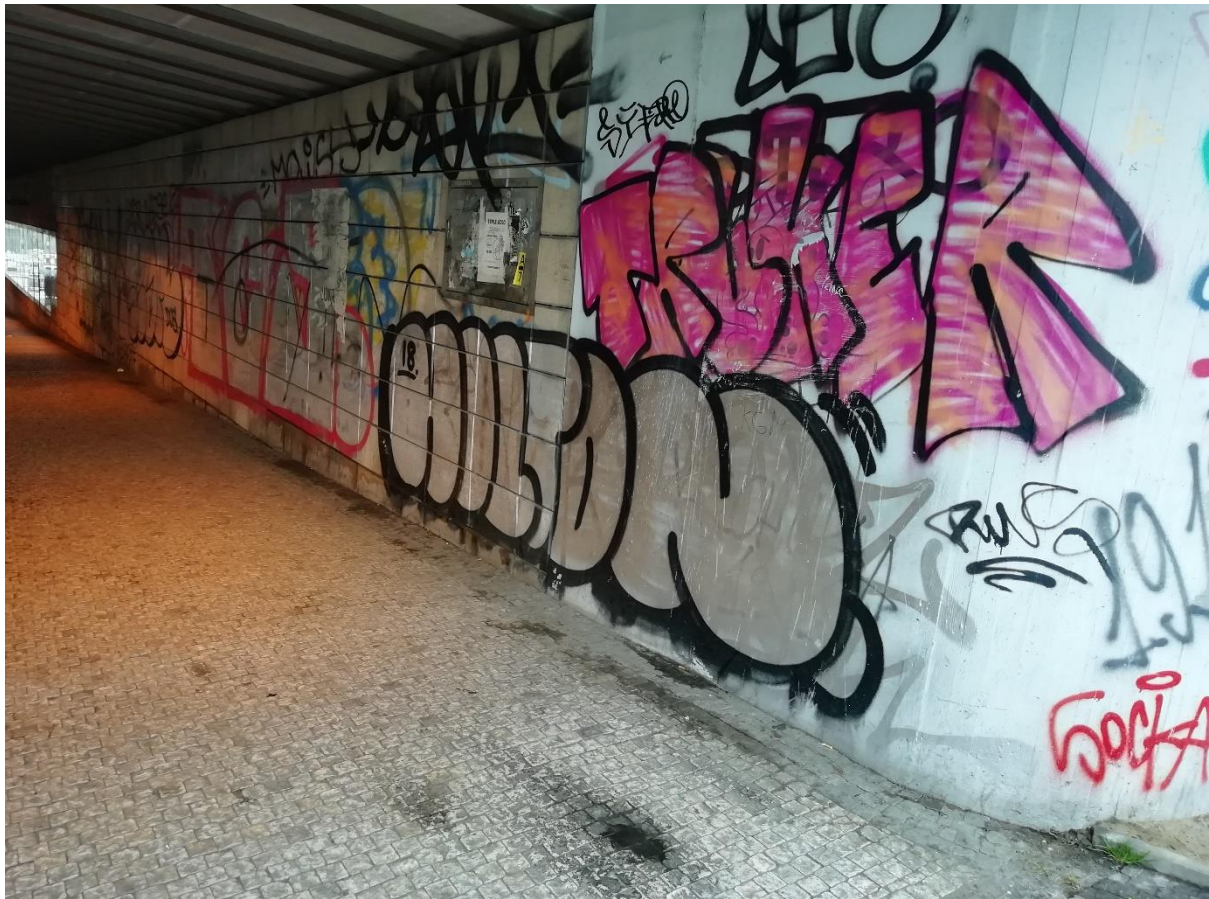
Figure 4.8: Showing graffiti under a bridge at Seifertova street, Prague 3
