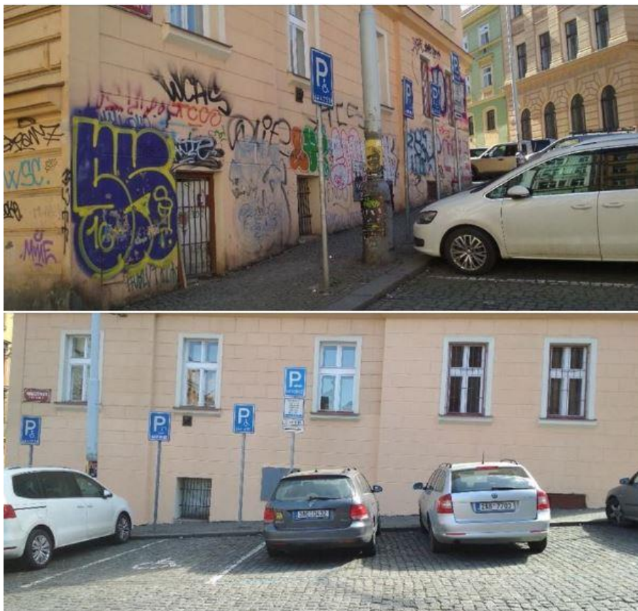
Figure 4.18: Showing a building restored from graffiti Source: (Antigrffiti program Prahy 3, 2018)
