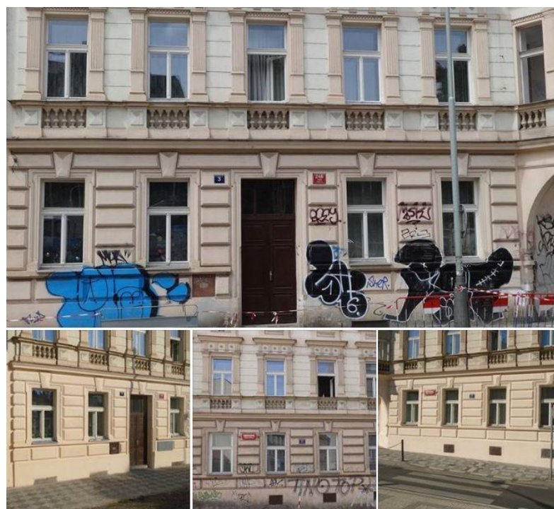
Figure 4.16: Showing a building restored from graffiti Source: (Antigraffiti program Prahy 3, 2018)
