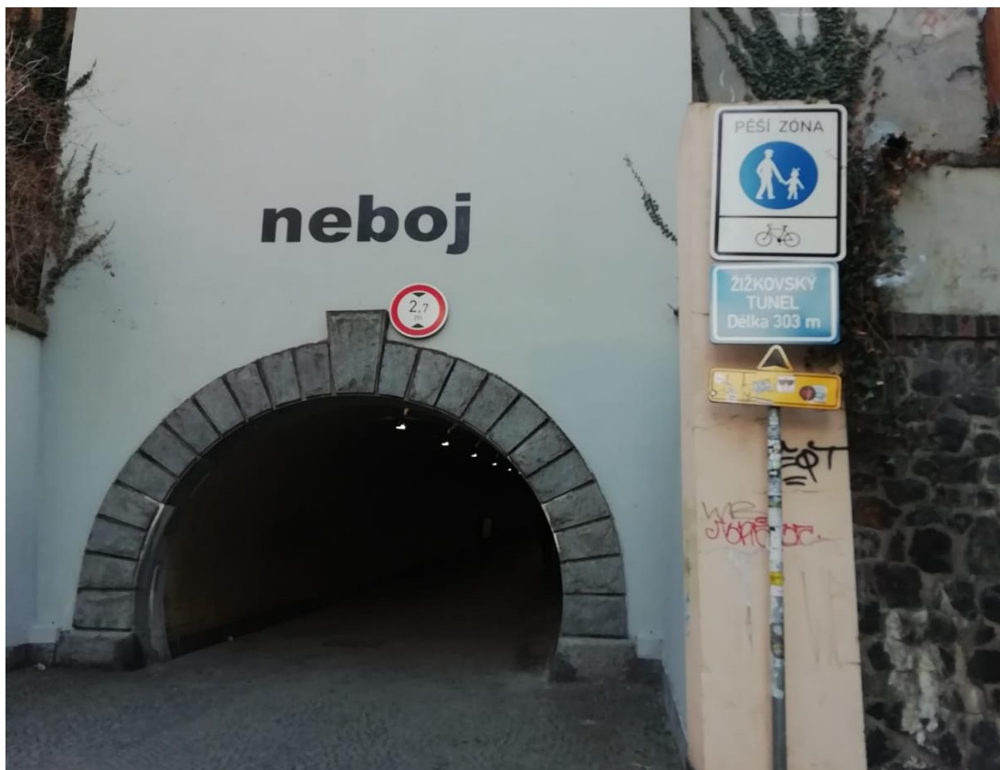
Figure 4.10: Showing Zizkovsky tunnel's entrance from Karlin
