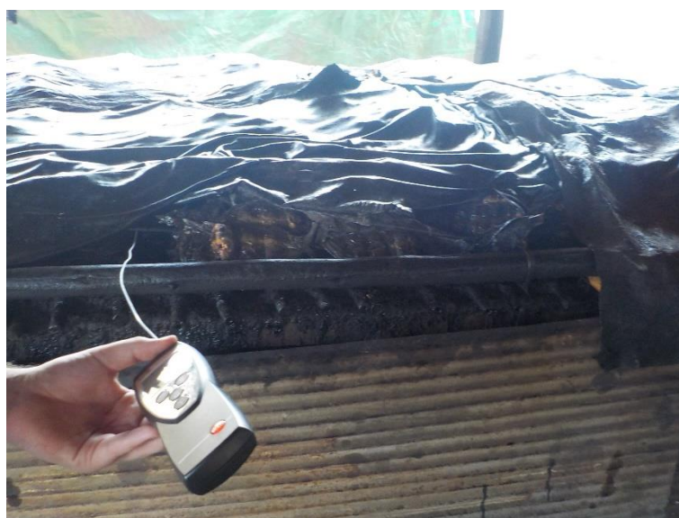
Figure 34 Temperature measurements, Tonlé Sap area, Cambodia.
