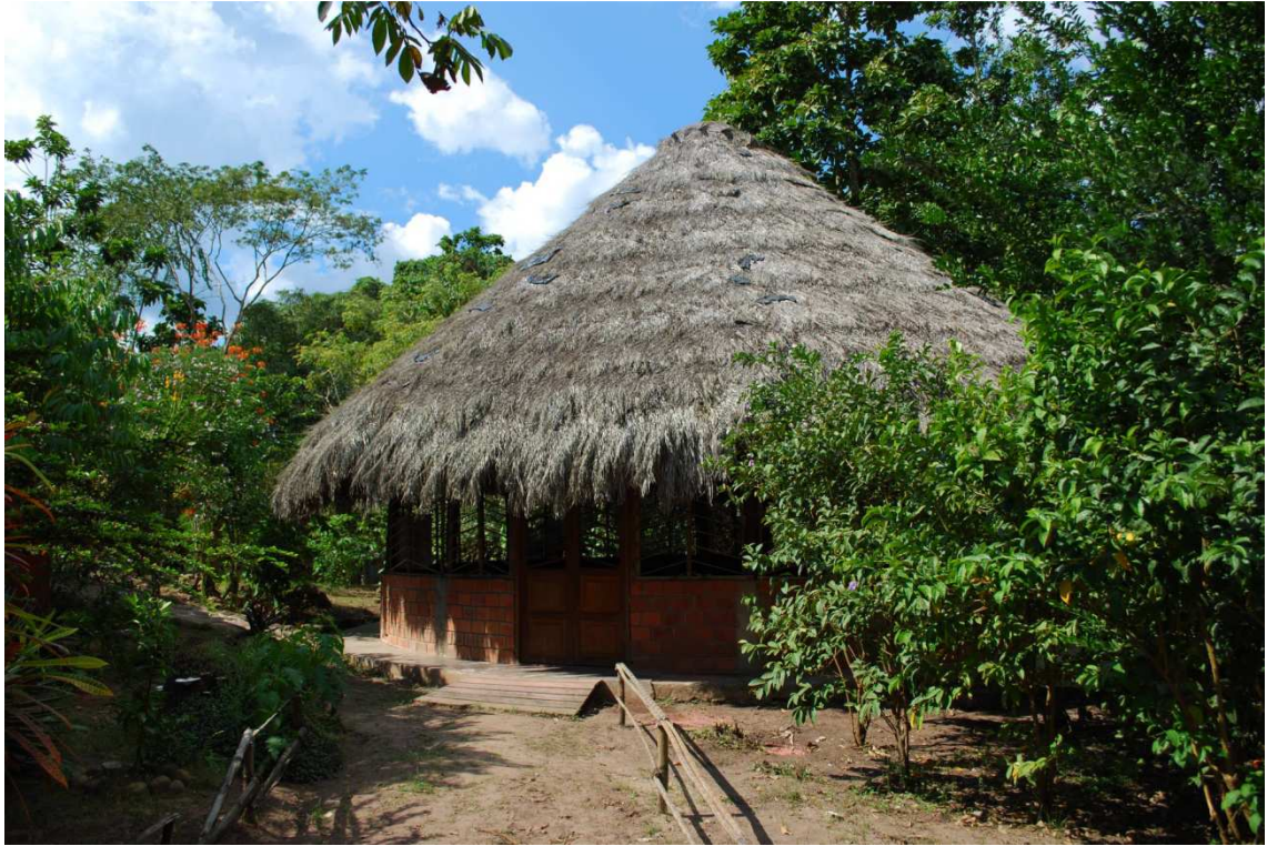
Fig. 4 TC Takiwasi in Peru – Maloca Chica, building designed for detoxification
