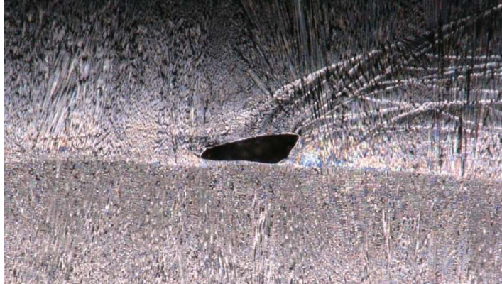
Fig. 52 Detail of crack between layers
