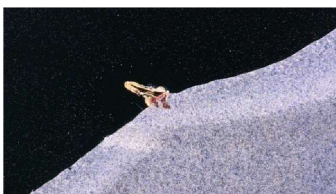
Fig. 44 Detail of crack I
