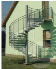
Figure 3.5: Stairs type Spiral
