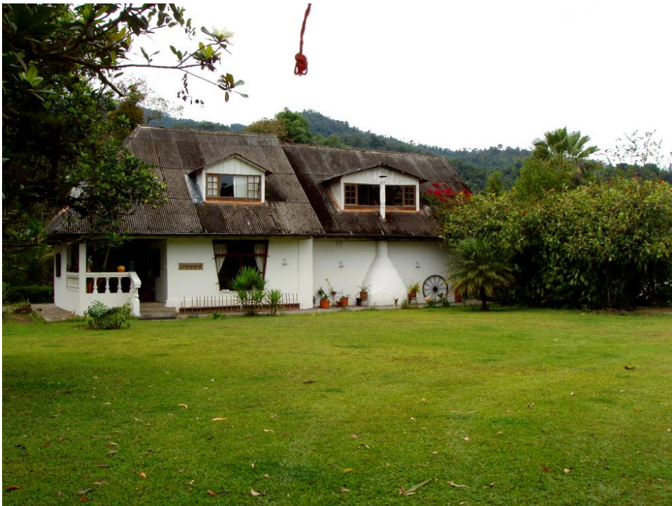
Annex 4 The main building of La Hesperia Biological Station & Reserve. Pichincha province, Ecuador
