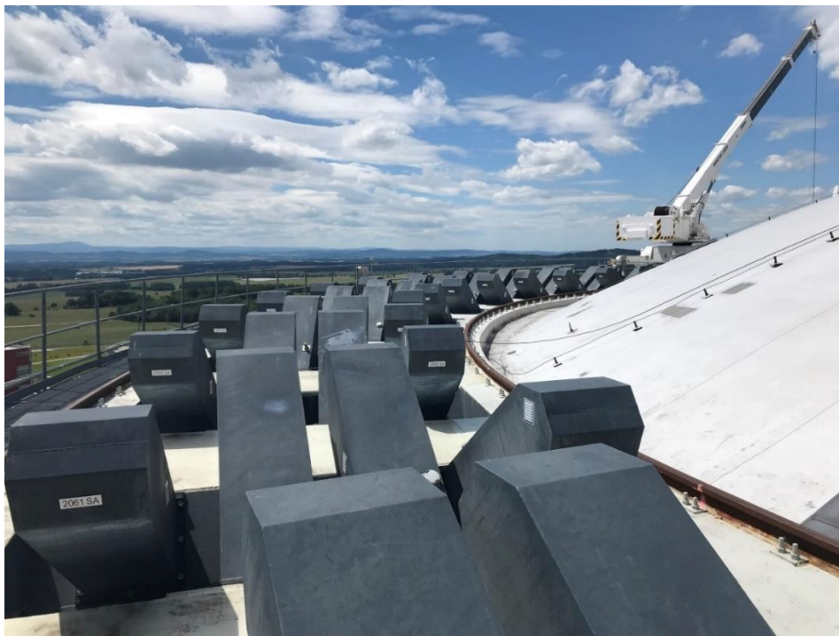
Figure 7. Ends of the pre-tightened ropes. Reprinted from Sviták (2020, November 13).
