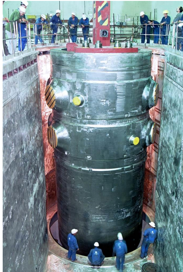
Figure 6. Pressure vessel. reprinted from ČEZ, a.s. (n.d.b).
