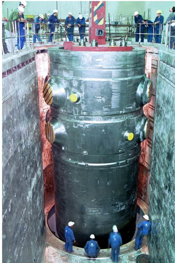
Figure 6. Pressure vessel. reprinted from ČEZ, a.s. (n.d.b).
