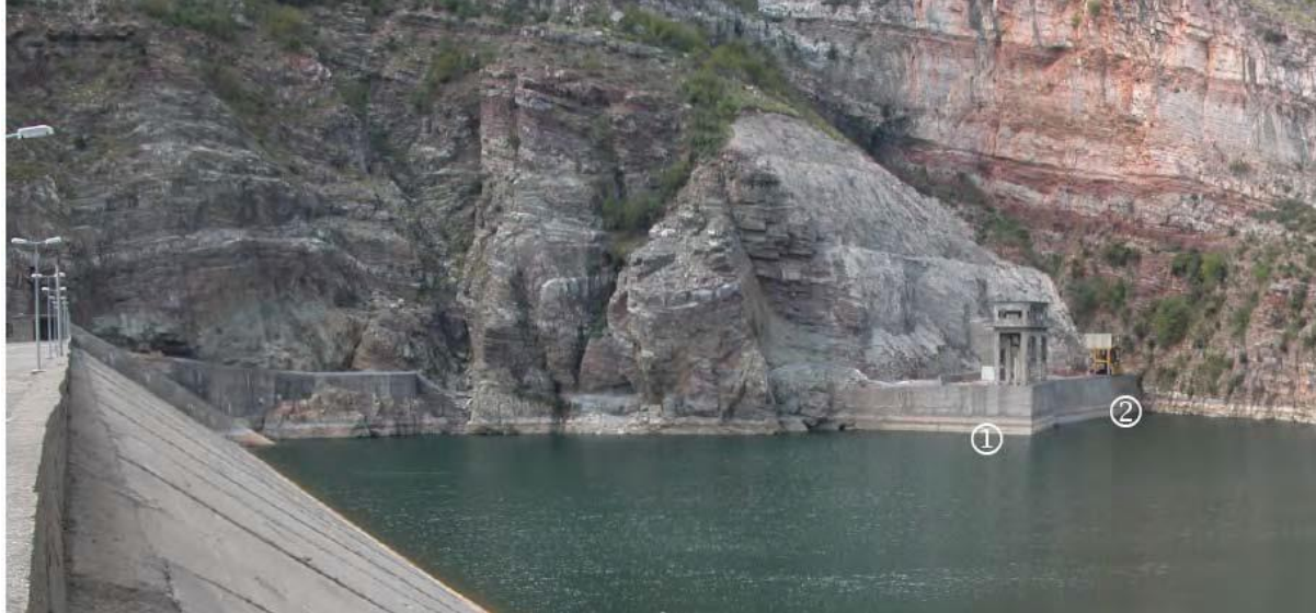
Fig. 4 Gate tower of the spillway No 4 (1) and power intakes (2)
