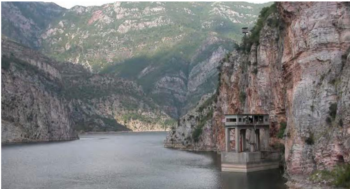
Fig.6 Intake tower of the spillway No 3
