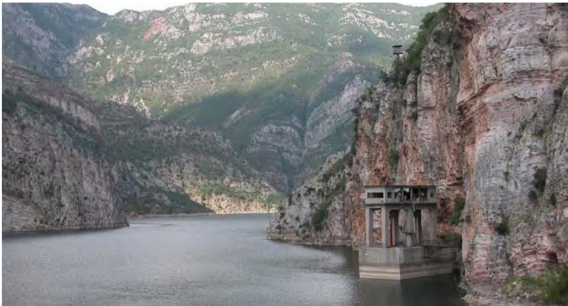
Fig.6 Intake tower of the spillway No 3
