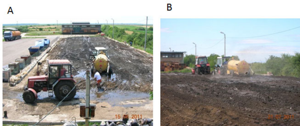
Figure 4.2: A: Preparation of bioremediation bio-pile. B: Bio-pile inoculation and biostimulation.
