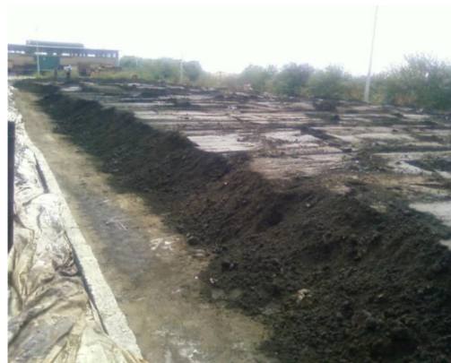
Figure 3.10: Bioremediation bio-pile.
